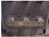
Typical UL test setup
